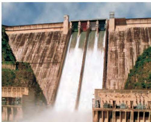
Bhakra Nangal Dam
